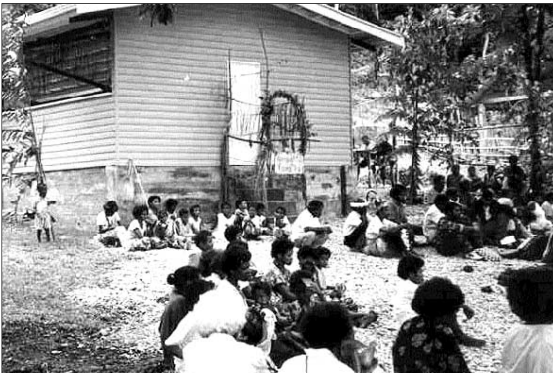
Community hall built by a mine-managed tax-credit scheme, Misima Island, Papua New Guinea
