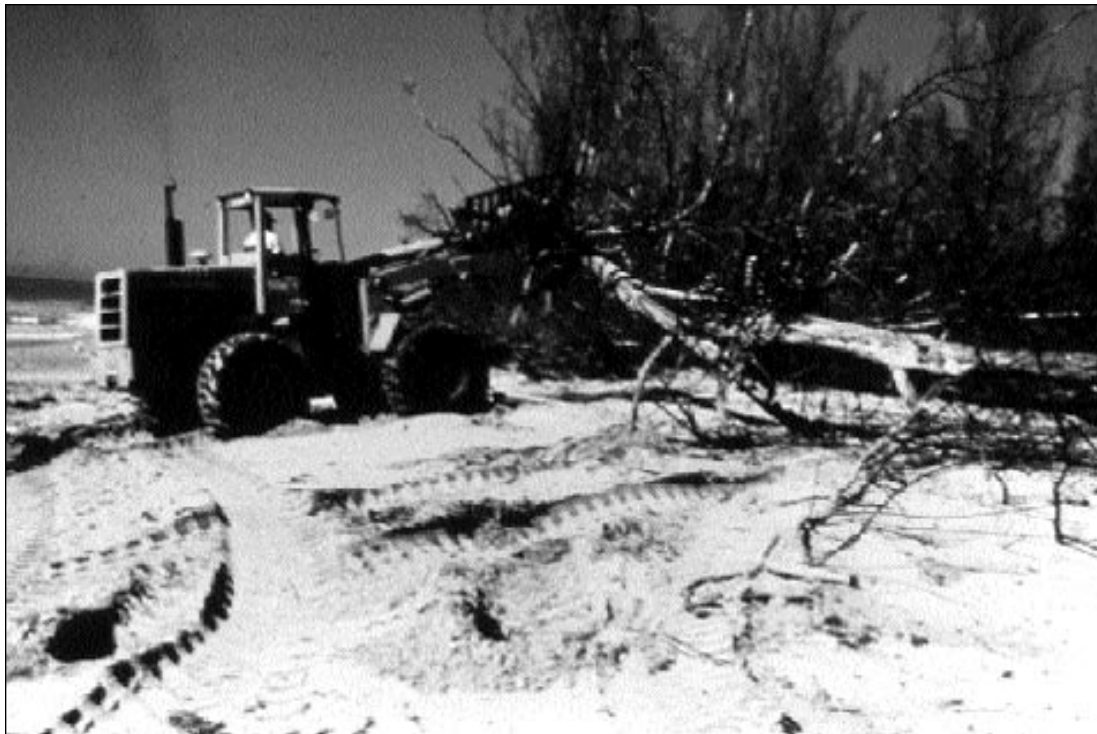
Clearing mangrove forest for development.
